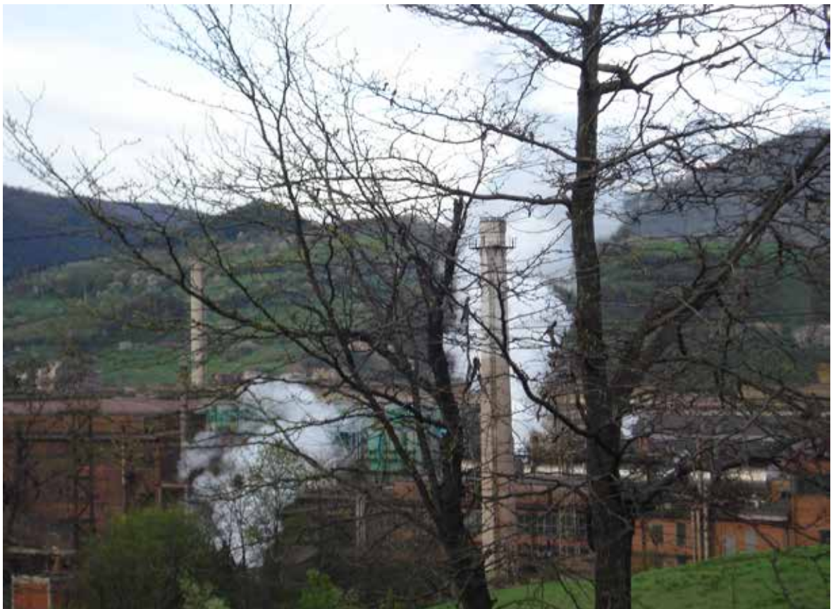
Arcelor Mittal, Zenica, Bosnia and Herzegovina
